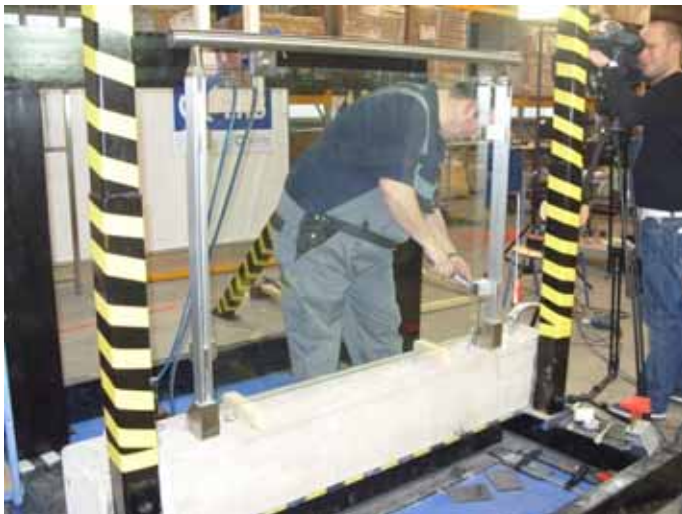
Photograph 6 Quickrail system during setup
